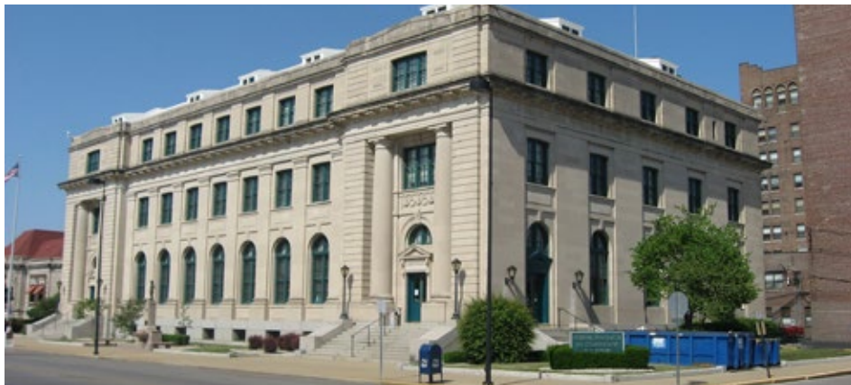
Danville US Post Office & Courthouse - Vermilion & Madison
